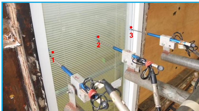
Photo 2: Location of transducer points on mock-up test specimen (View from inside building)
